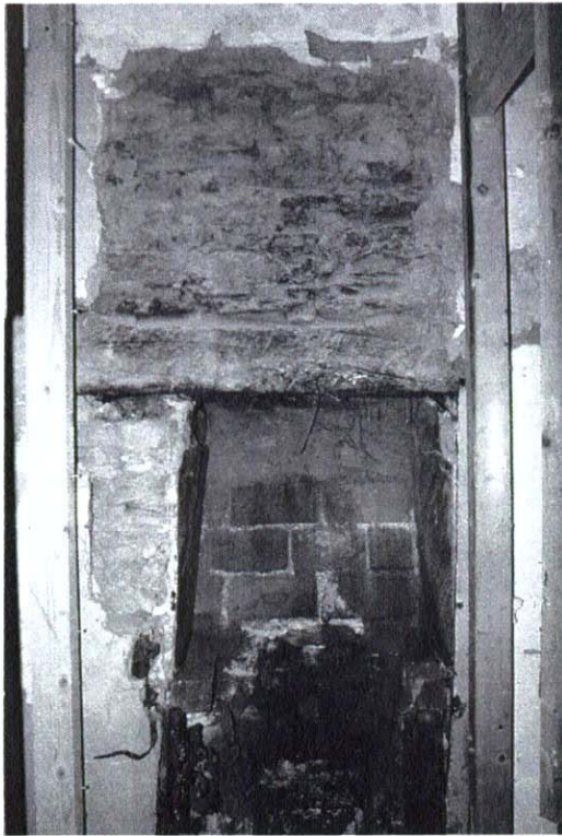
Plate 5 1 st -floor RH room (fireplace with inverted lintel). Chamfered oak lintel with tongue stops, now upside-down, probably re-used when fireplace was remodelled.
