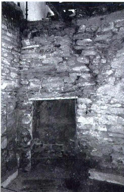
Plate 20 1 st floor LH room (rear wall, fireplace). Note rebuilt walling surrounding fireplace.
