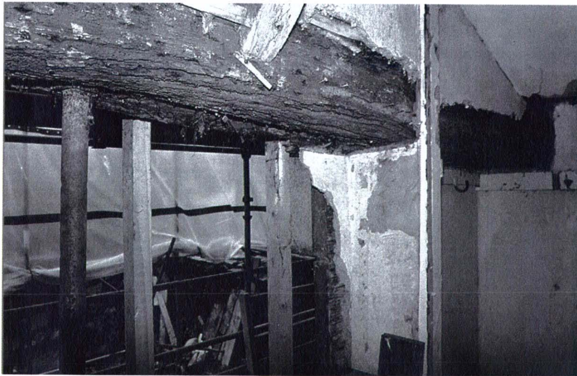
Plate 32 Rear wall (beam linking walls and supporting roof in staircase area).
