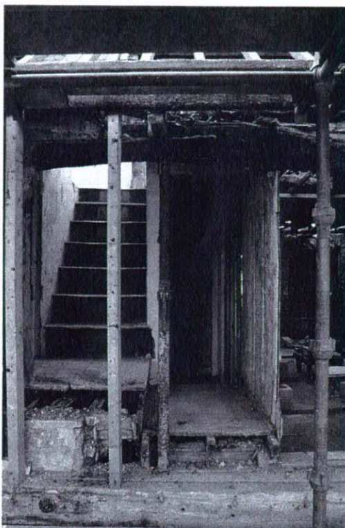
Plate 31 Stairs to 1 st -floor level. Note muntin and plank partition right of stair passage.
