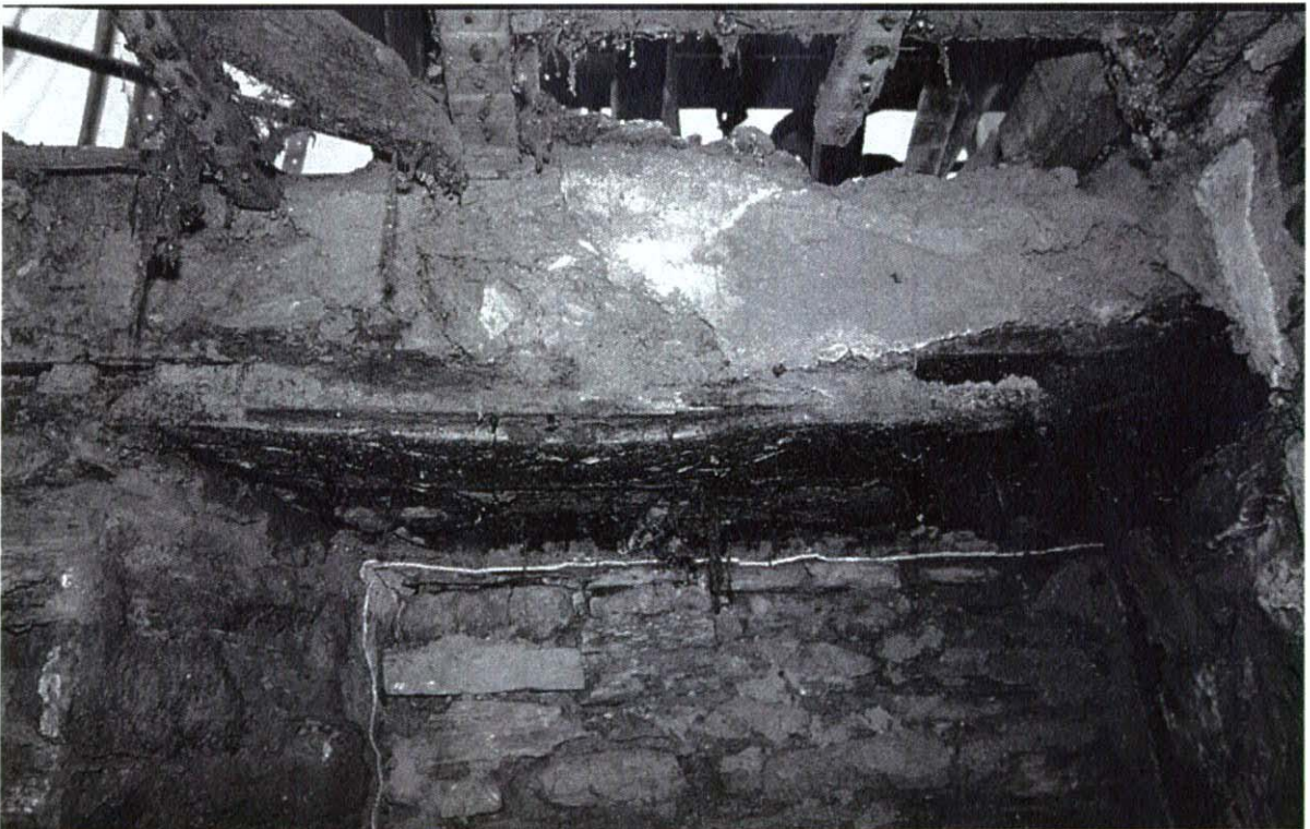
Plate 18 1 st floor LH room (NE corner showing blocked window and re-used roof timber). Re-use of collar from 16 th century arch-braced roof structure.
