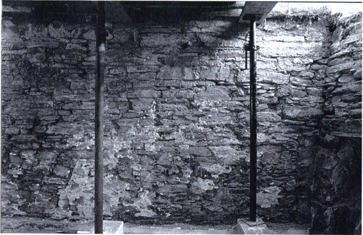
Plate 19 1 st floor LH room (E wall including rebuild on right to include chimney)
