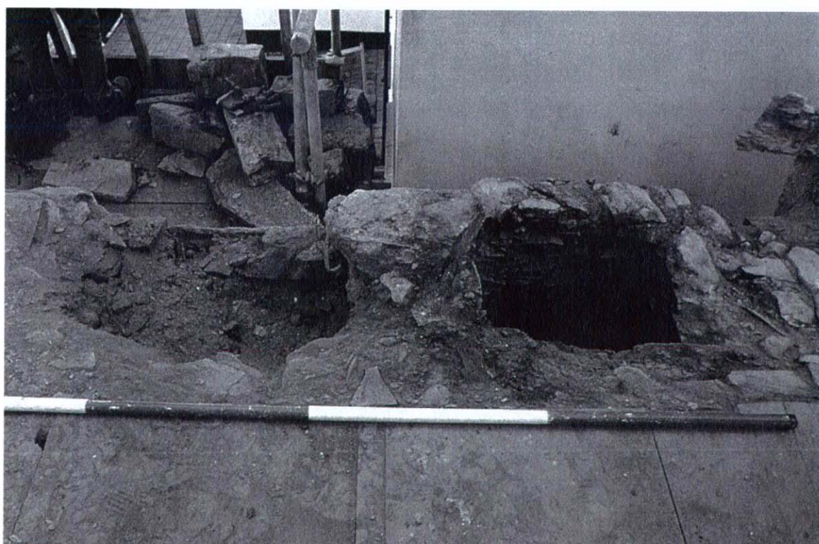
Plate 24 E gable end wall (flues to attic floor level). Both flues for adjacent former house prior to demolition and rebuilding of outer skin of flues.
