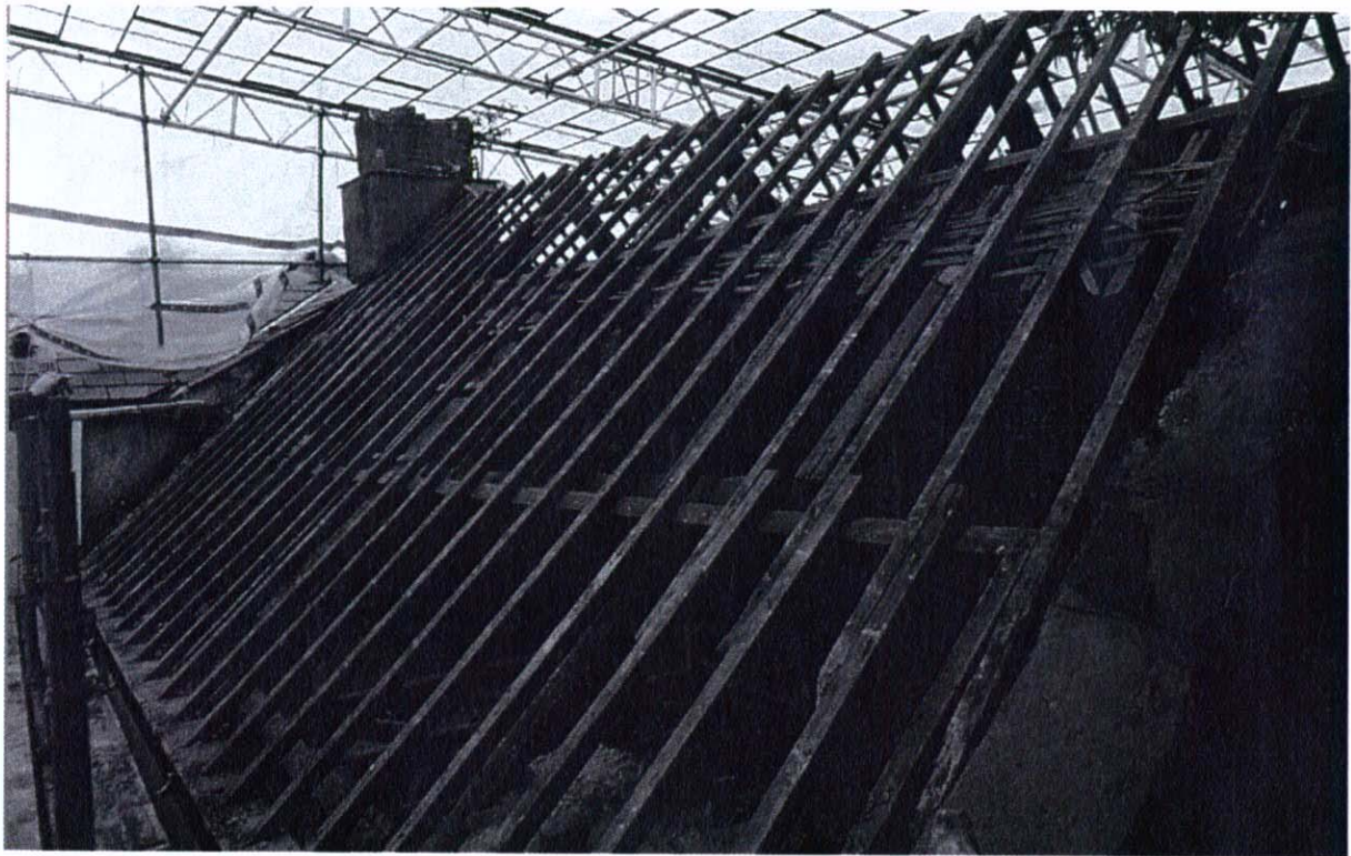
Plate 35 Roofline towards west (chimney stack prior to demolition + scaffolding protection system)
