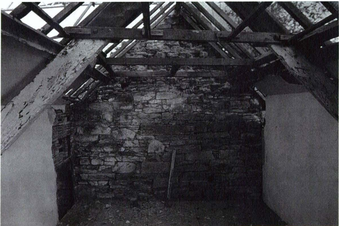
Plate 22 E gable (interior prior to demolition). Note good quality rubble masonry (but leaning outwards due to failed structure underneath)
