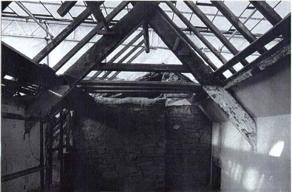
Plate 25 W gable. Unstable stone stack removed.
