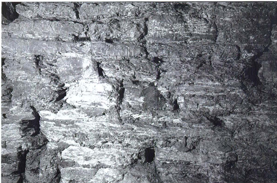
Plate 9 Ground floor E wall (tooling on stones). Generally well constructed and tooled rubble masonry reinforcing opinion about an early date.
