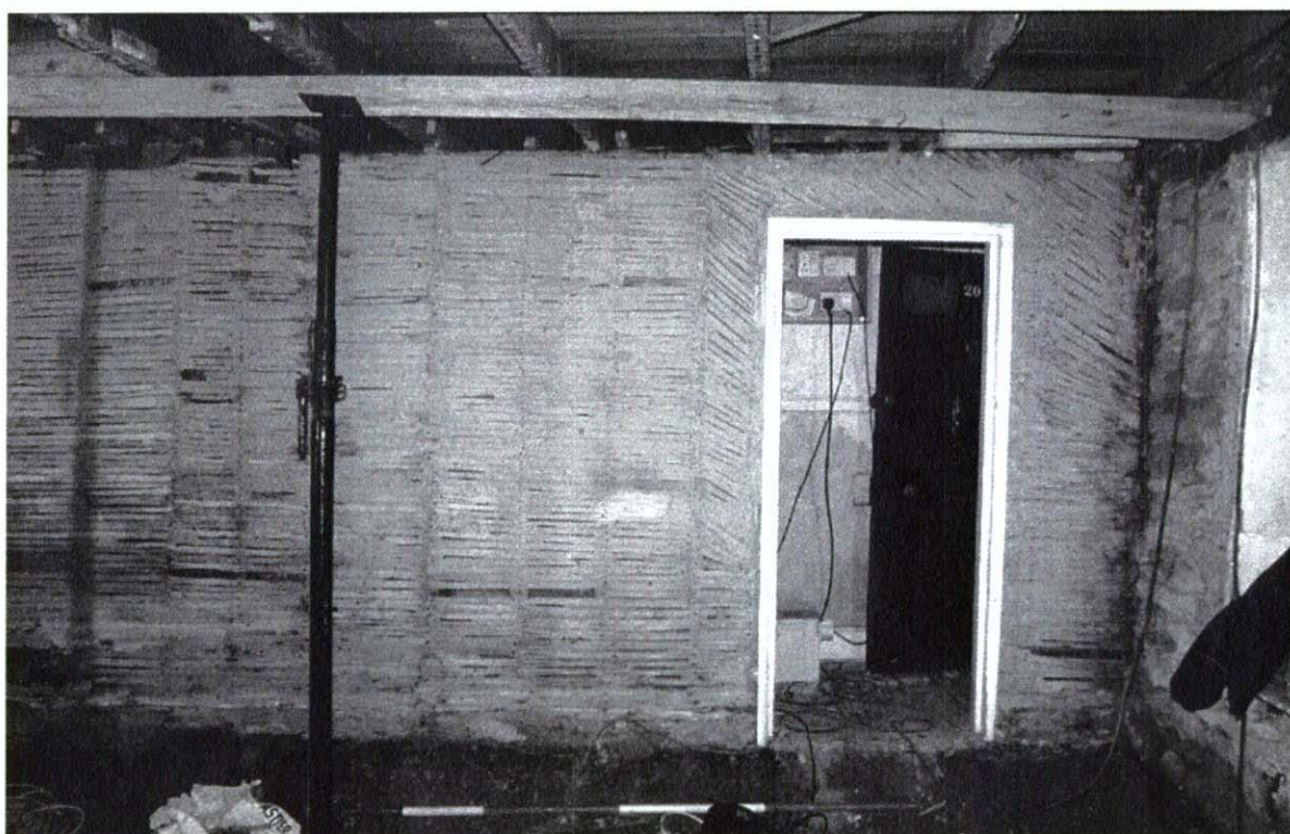
Plate 10 Ground floor LH room (lath construction of internal partition c1800). Good example for use of regular split-lath lengths generally but also using some diagonally set laths.
