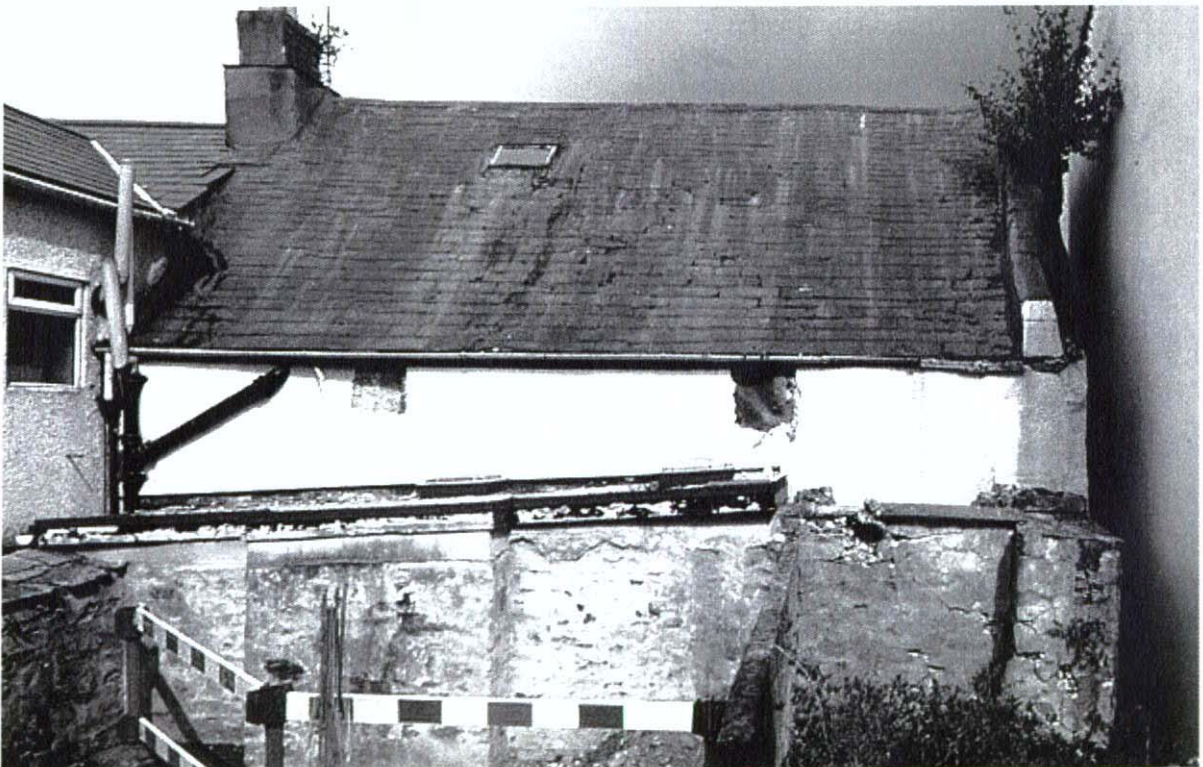
Plate 2 Rear elevation (pre works). Remains of former cottage in foreground; rendered rear wall; rag slate roof coated with bitumen; rendered stone and brick stack.
