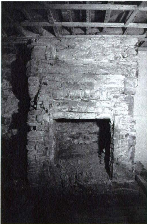
Plate 14 Ground floor RH room (principal fireplace partly opened up).
