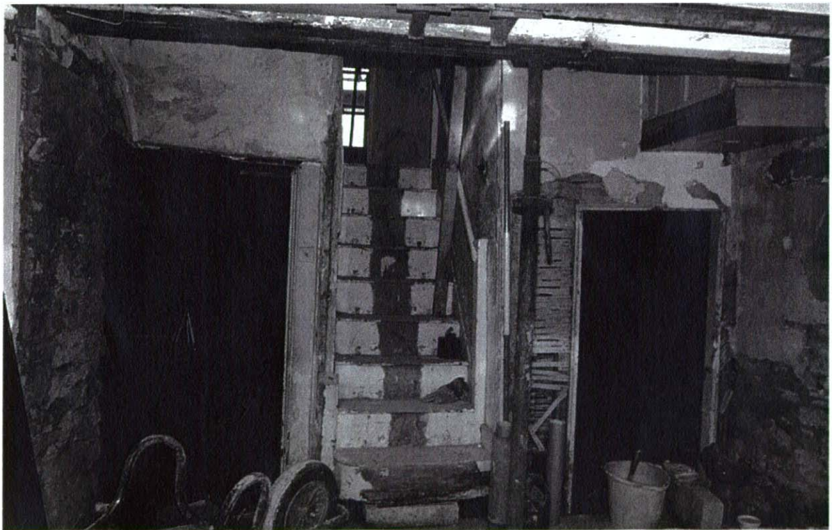
Plate 30 Stairs to ground-floor level. Note thick masonry walls at left and right.
