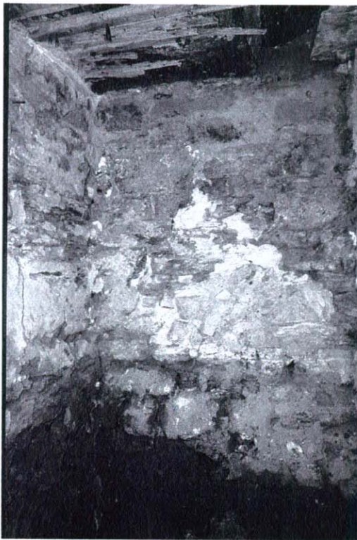
Plate 15 Ground floor RH room (recess at SW corner). Probable former window opening with lime plaster visible in the splayed jambs.
