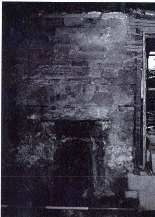
Plate 8 Ground floor LH room (S wall showing fireplace). Original oak lintel removed and size of fireplace reduced in the 19 th century. Foundation shallower than that of E wall.
