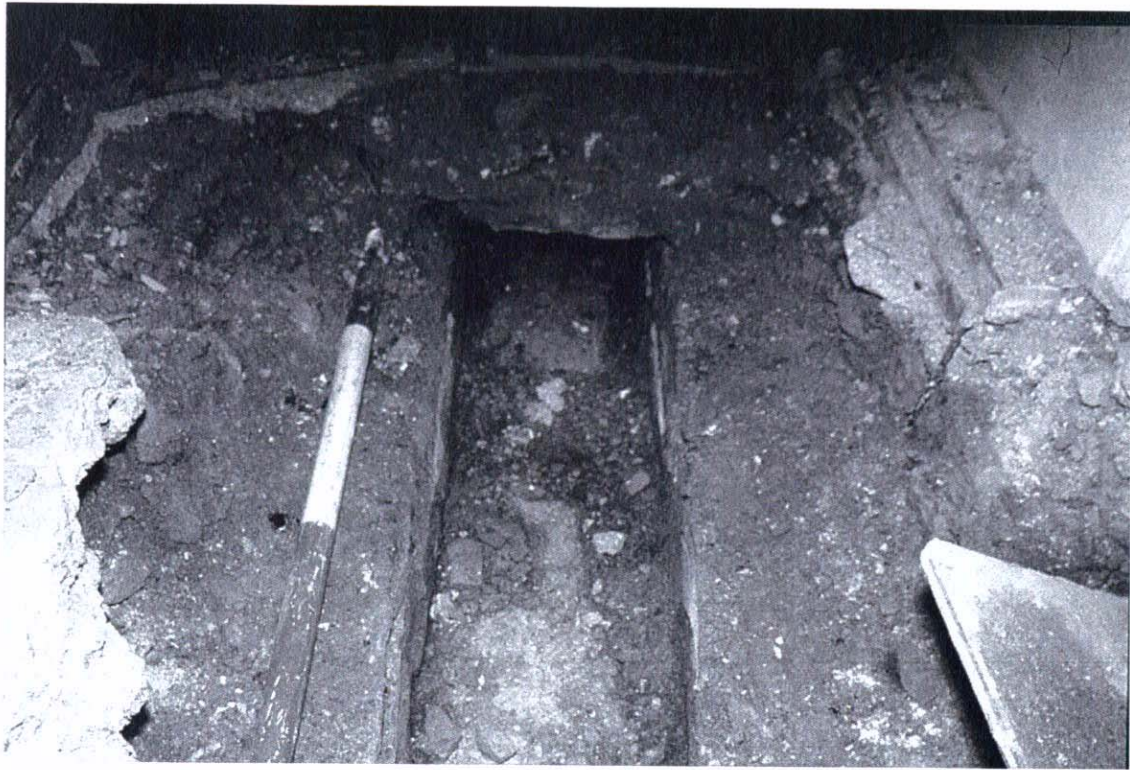
Plate 11 Entrance hall (slate land drain revealed under c1900 tiled floor). Unusual feature but similar drain found recently at Manaccan former vicarage.
