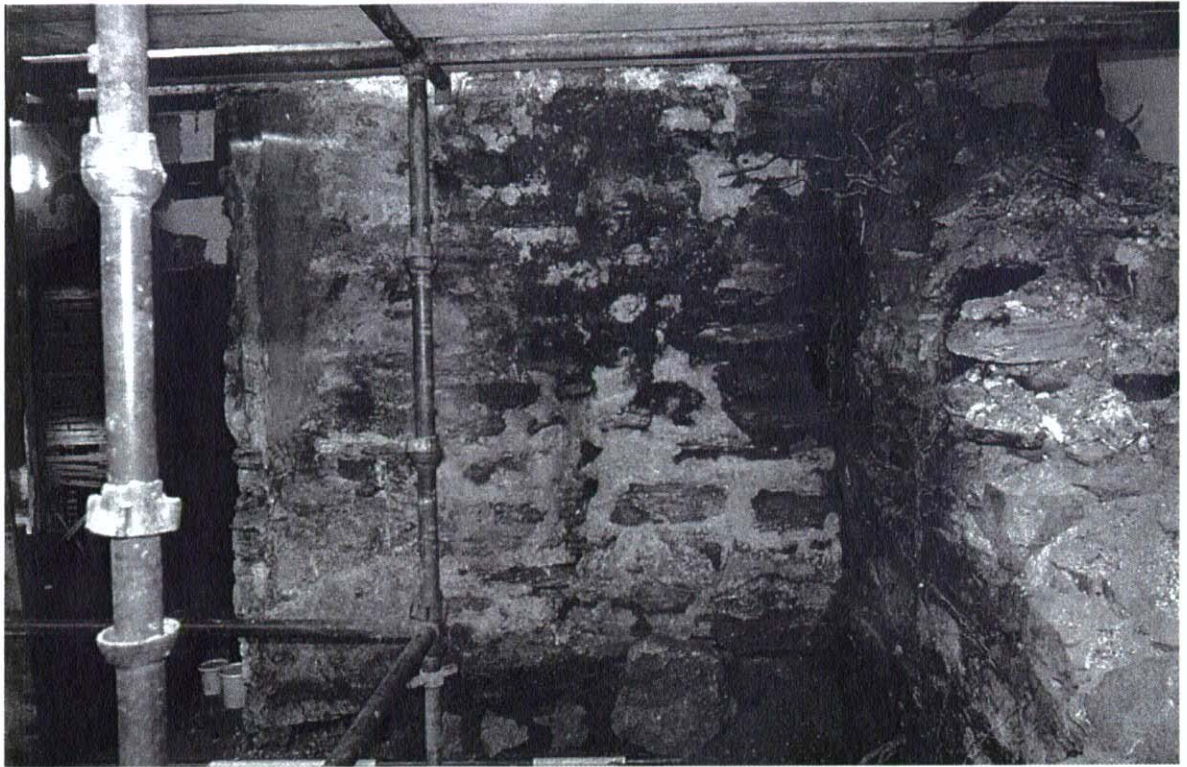
Plate 33 Ground floor rear wall adjacent to SE corner (extent of wash house of No 20 feeding to flue of back kitchen of former No 18).
