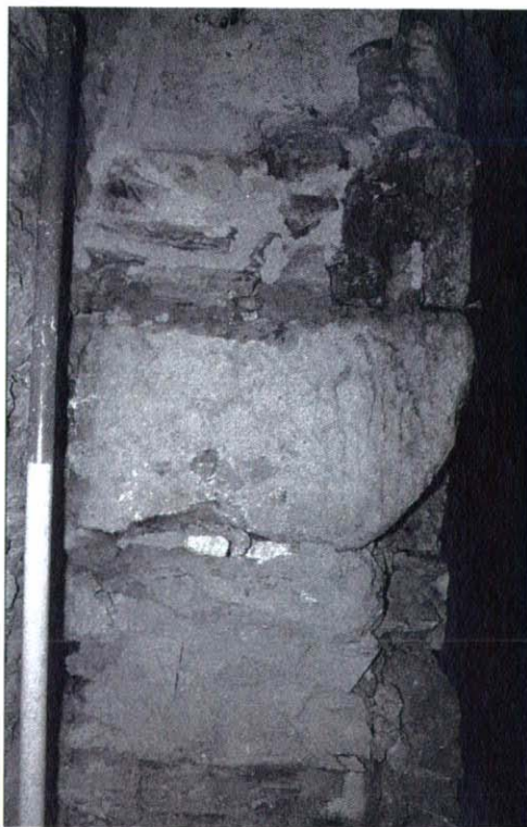
Plate 16 Principal fireplace LH return (granite corbel and oak lintel end with old mortise indicating re-use).
