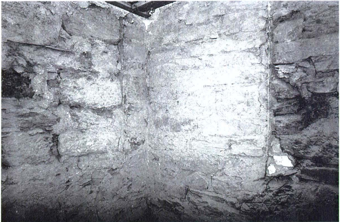
Plate 21 1 st floor RH room (blocked opening in SW corner). Blocked window opening.
