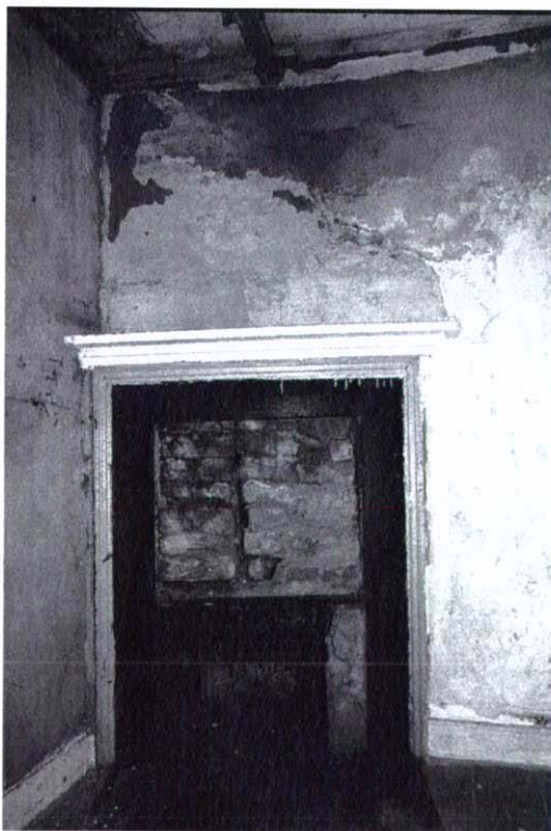
Plate 4 1 st -floor LH room. (c1800 chimney-piece). Simple moulding and moulded shelf suggests a late 18 th or early 19 th century date; simple hobs and grate.
