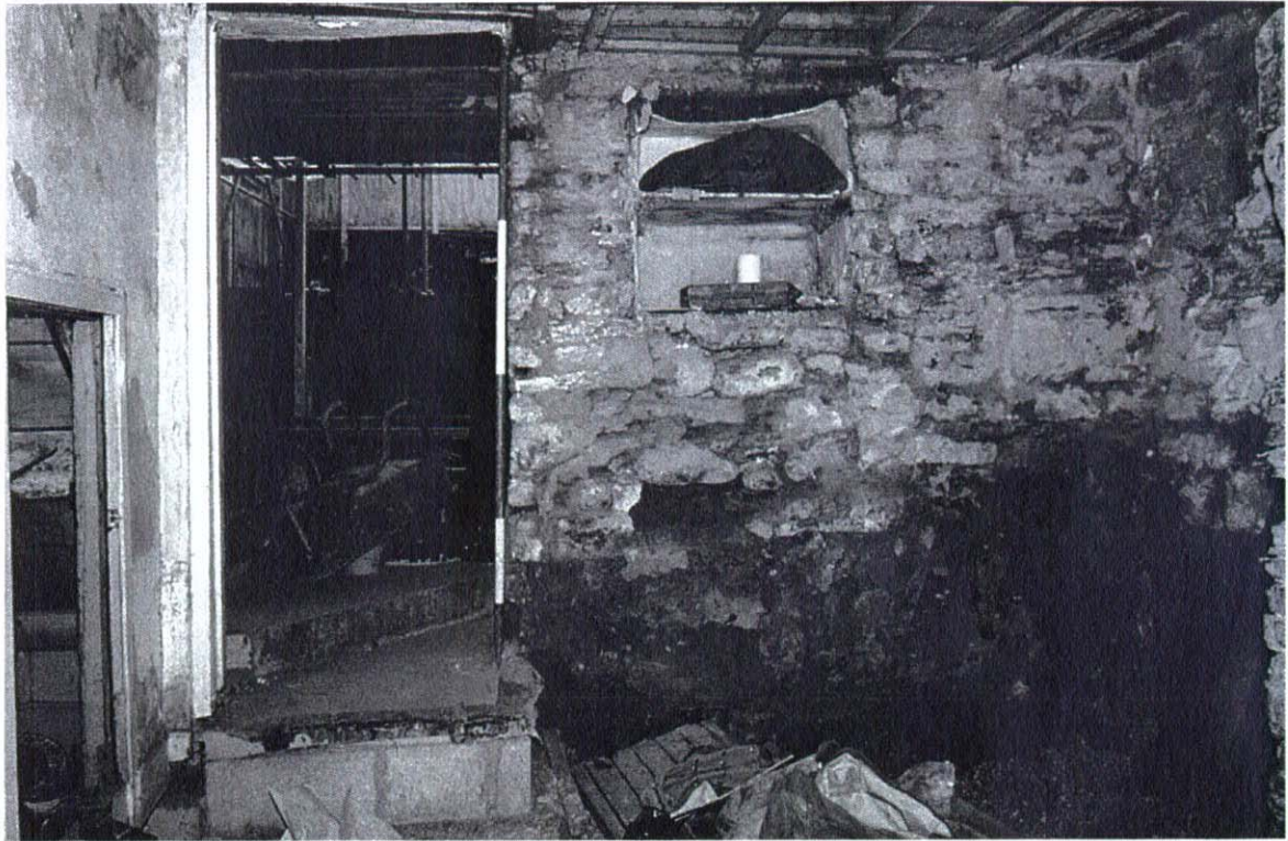
Plate 13 Ground floor RH room (S wall with foundations and keeping place). Very high foundations indicate build method on a sloping site. Most of wall probably 18 th century.
