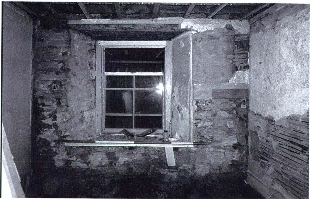
Plate 12 Ground floor RH room (N wall: altered window openings; joist sockets for earlier 1 st floor, and support for former wooden ground floor).
