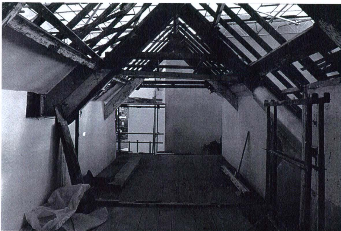
Plate 23 E gable (post demolition). Note roof structure and floor construction.
