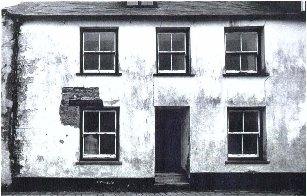
Plate 1 Front elevation (pre works). 20 th century cement-based render resembling stucco with incised lines to resemble ashlar; re-used oak lintel revealed as part of enabling works.
