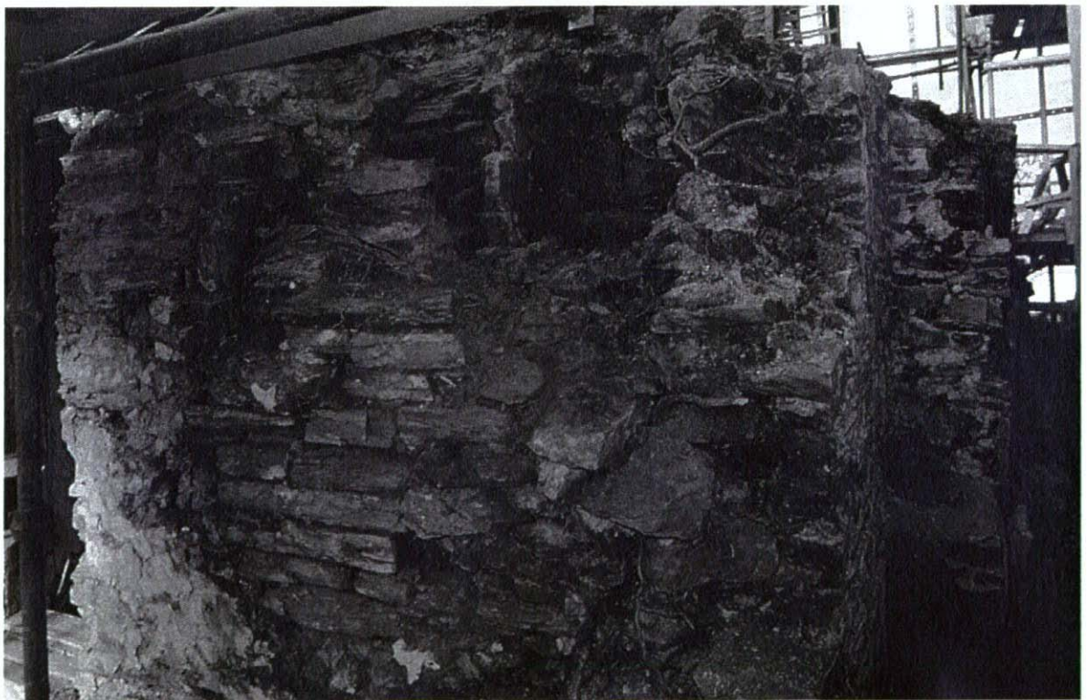
Plate 34 Exterior SE corner (remodelling phases and flues).
