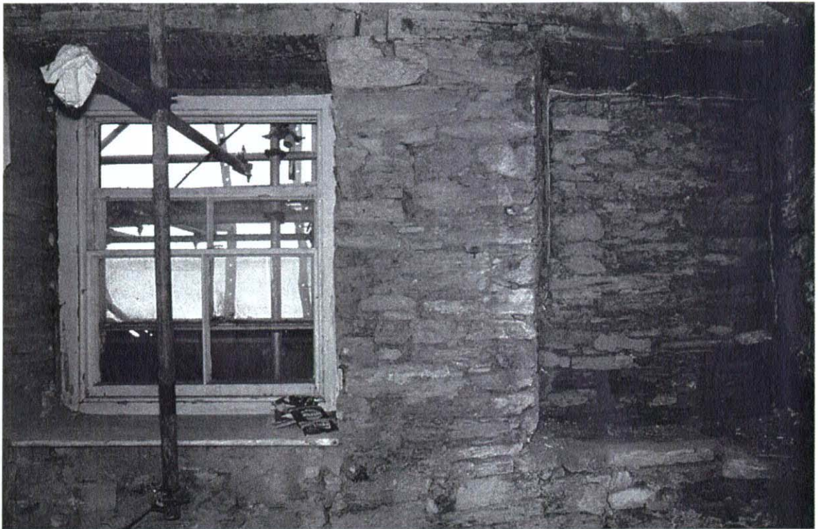
Plate 17 1 st floor LH room (existing window and blocked window). Re-used oak lintels.
